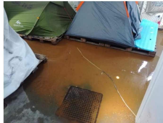
One of the more severe sewage leaks we have seen, on Level Three
