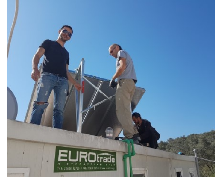
Installing a new solar boiler unit
