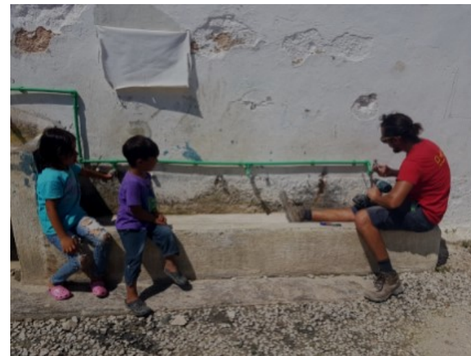
Replacing taps on some outdoor sinks
