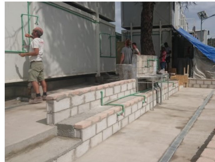
Adding showers to the camp's largest wash pad
