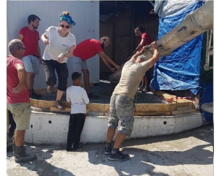
Pouring concrete for a new wash pad
