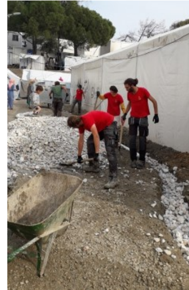
Shovelling gravel to build a French drain
