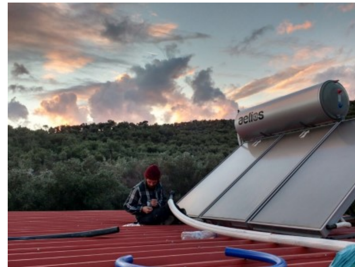
Insulating hot water pipes
